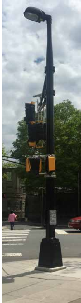
Pedestrian lighting on traffic signal posts
