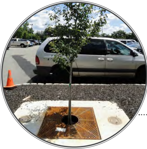
LOCATION: Parsippany, NJ This enhanced tree pit is located at the Parsippany-Troy Hills Municipal Court parking lot. The tree pit collects and filters water from the existing parking lot.
