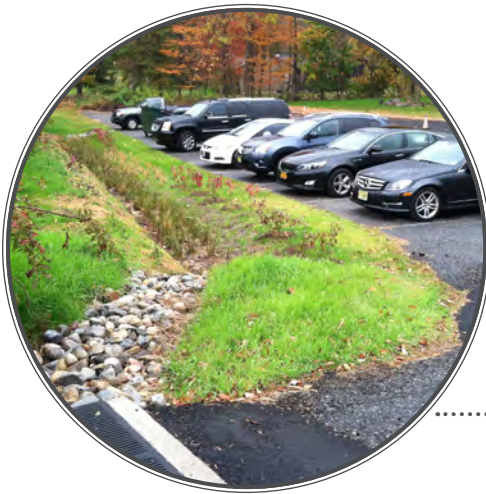
LOCATION: Parsippany, NJ This bioswale was installed at St. Gregory's Church. The bioswale was designed to capture water from the parking lot and move it toward the forest area on the south end of the site.
