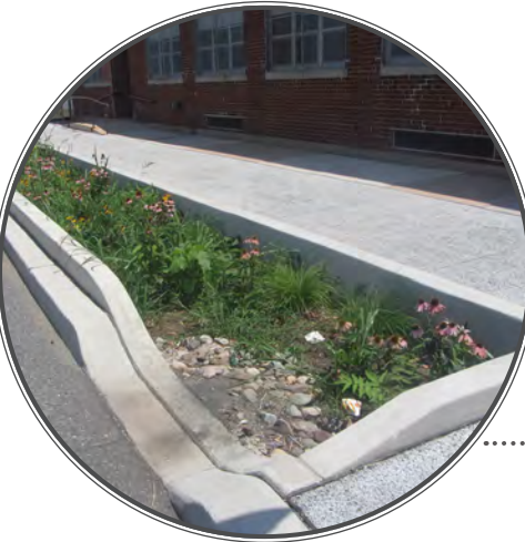
LOCATION: Camden, NJ This stormwater planter was designed to capture stormwater runoff from the street in front of the Brimm School in Camden, New Jersey.
