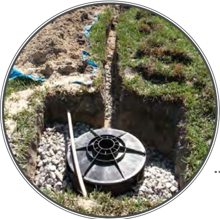
LOCATION: Holmdel, NJ. This residential dry well was installed in Monmouth County. It is a underground system that uses an empty container to store large quantities of stormwater during rainfall events.
