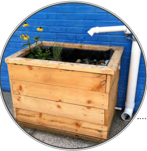
LOCATION: Camden, NJ Downspout planters are installed at the end of a downspout to capture, store, and slowly discharge stormwater back to the nearest storm sewer system.
