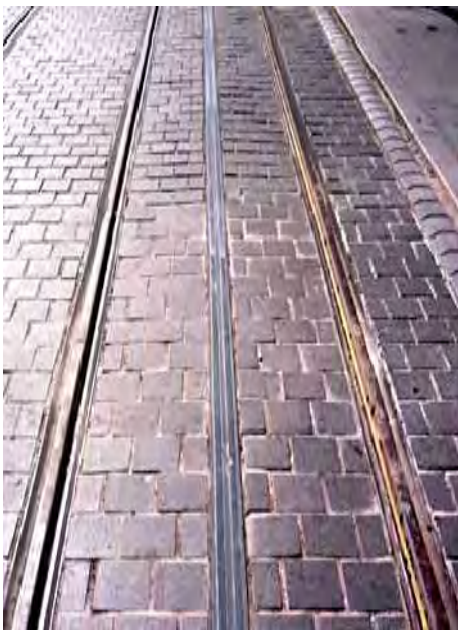
Figure 1-18 Bordeaux tracks with imbedded traction power
